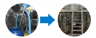
Instead of utilizing intermediate containers (pictured left) to hold product in between two stages of the production process, site engineers installed a pump that linked the fed product directly to the next stage, reducing water and cleaning chemical usage.
